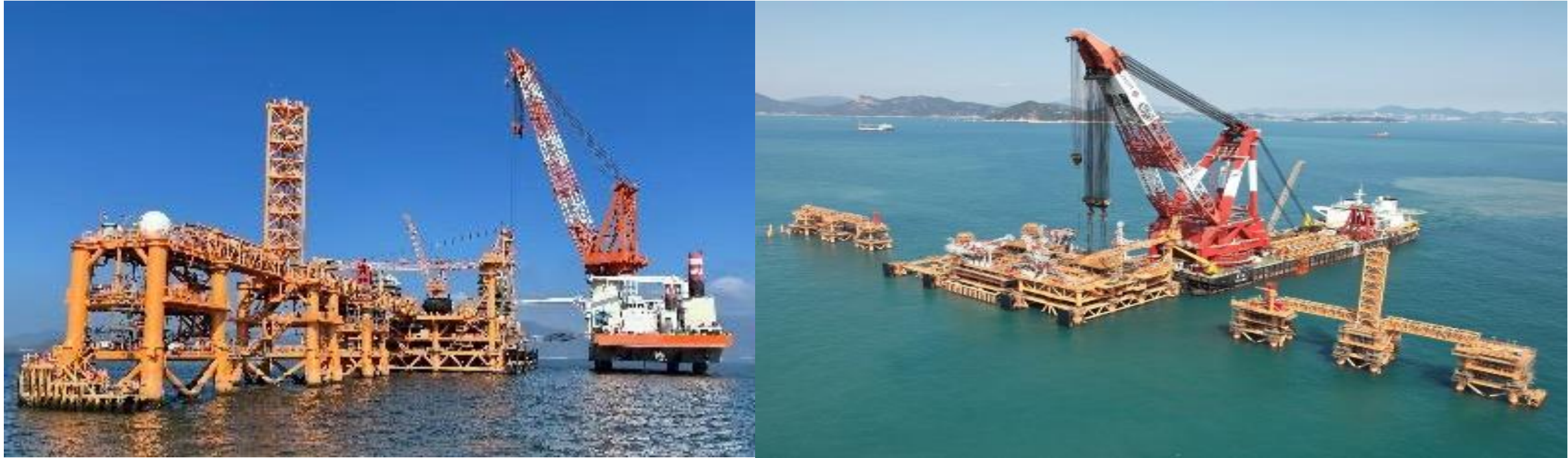
Topside Structure & Equipment Installation
