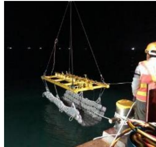
Rock Armour Placement
