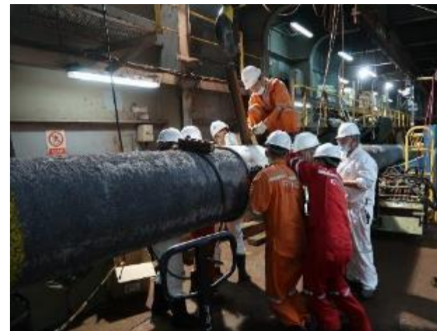
Welding of Line Pipes
