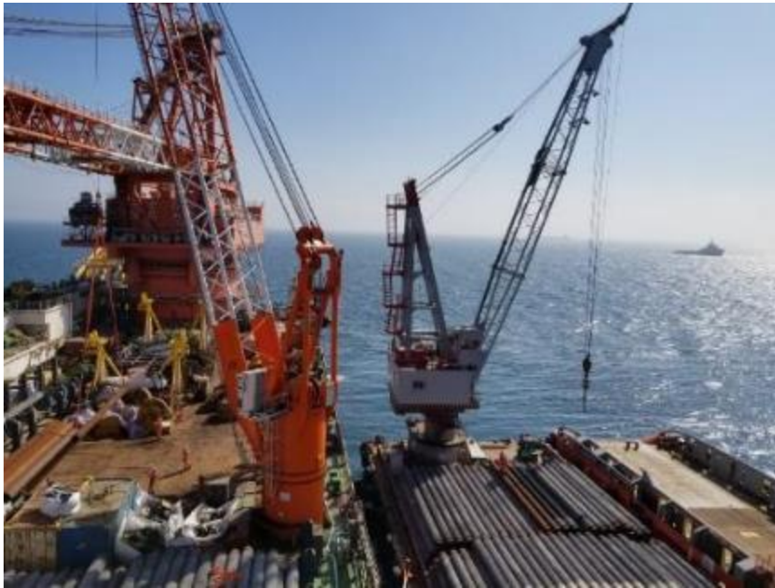
Supply of Line Pipes
