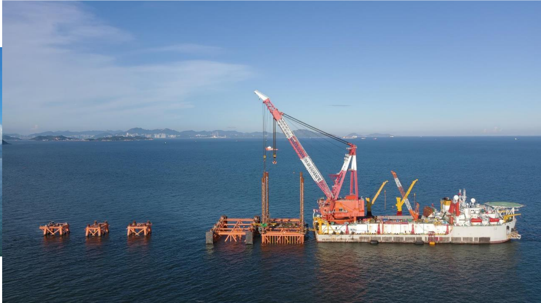
Jacket and Piling Installation
